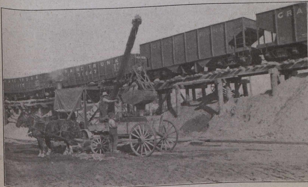
Unloading Aggregates with a Byers Hoist at Camp Borden.
