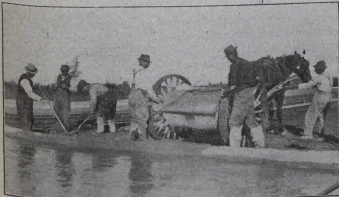
Fig. 4.—Concrete Being Hauled to Job in Carts.
