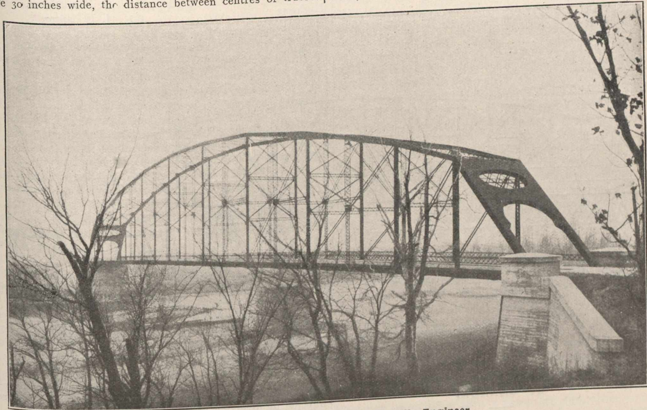
The Elizabethtown Bridge, H. C. Tyrrell, Engineer.
