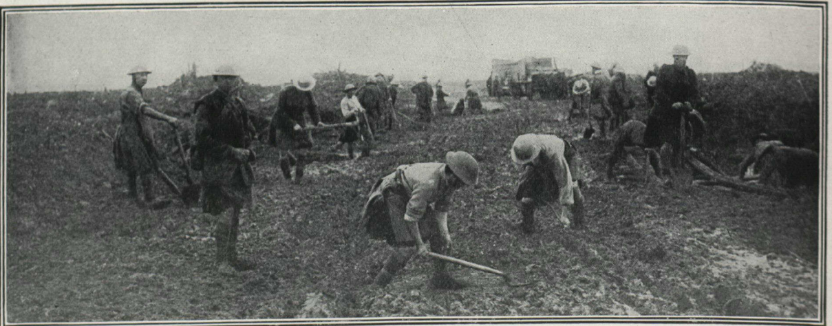
REPAIRING A ROAD TO COURCELETTE
