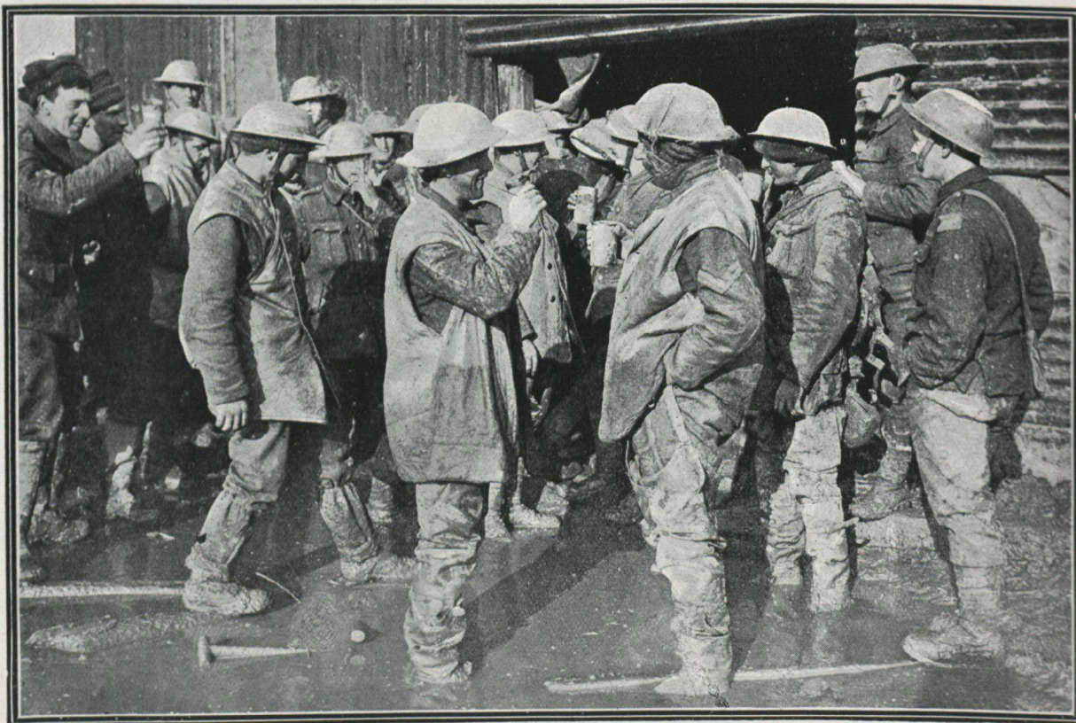
HOT COFFEE IS VERY COMFORTING AFTER THE TRENCHES
