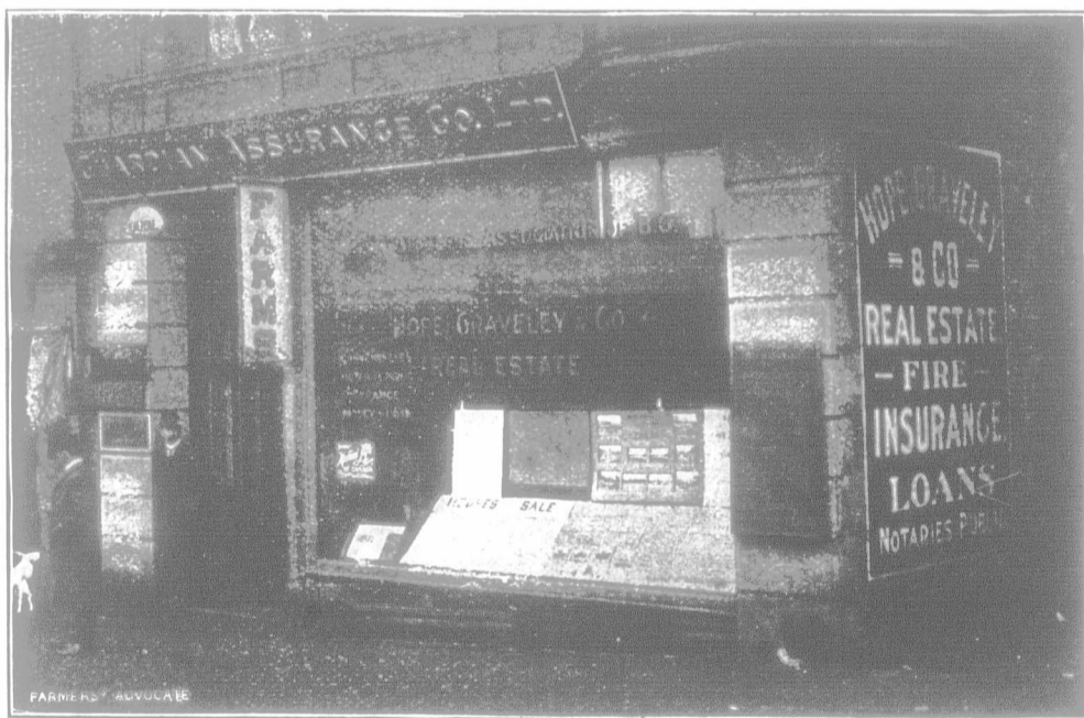
322 Cambie Street, Vancouver.
