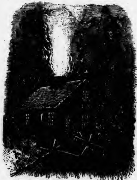
THE CHIMNEY ON FIRE.
