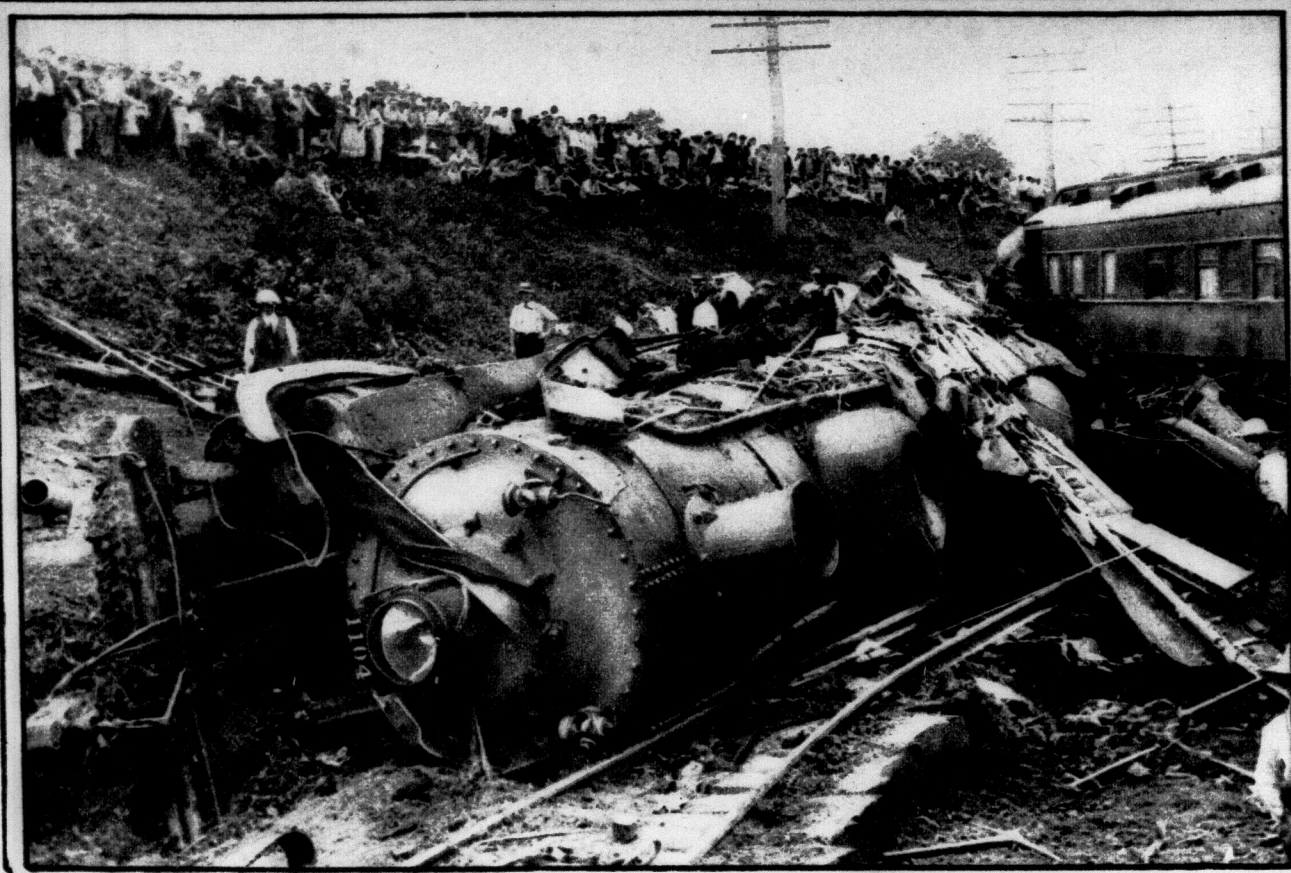
Seven killed, 100 injured when storm-clogged switch wrecks Delaware, Lackawanna and Western Railroad train at Rockport, New Jersey
