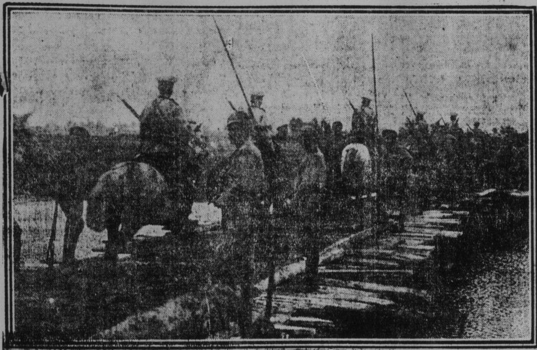
Russian mounted soldiers crossing hastily built bridge. Men on both sides are keeping the boards in position.
