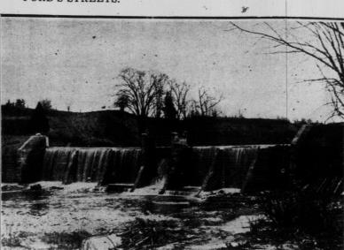
The first dam of the arc type to be built in Canada. It is the Milne dam at Berkely Lake, Markham, and it has backed up the water so that launches have now a clear run of three miles.
