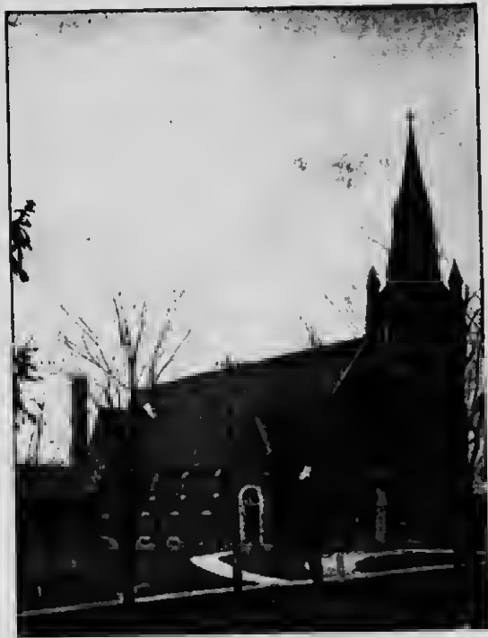
CATHOLIC CHURCH, OSHAWA
