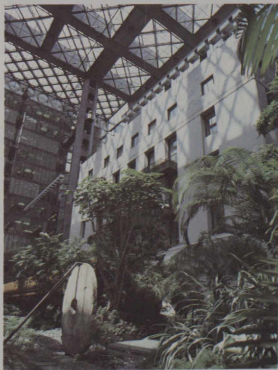
When the Bank of Canada outgrew its quarters in the early 1970s, architect Arthur Erickson designed two towers of glass and oxidized copper to flank the original stone structure. The three buildings are connected by bridges within an enclosed glass courtyard.
