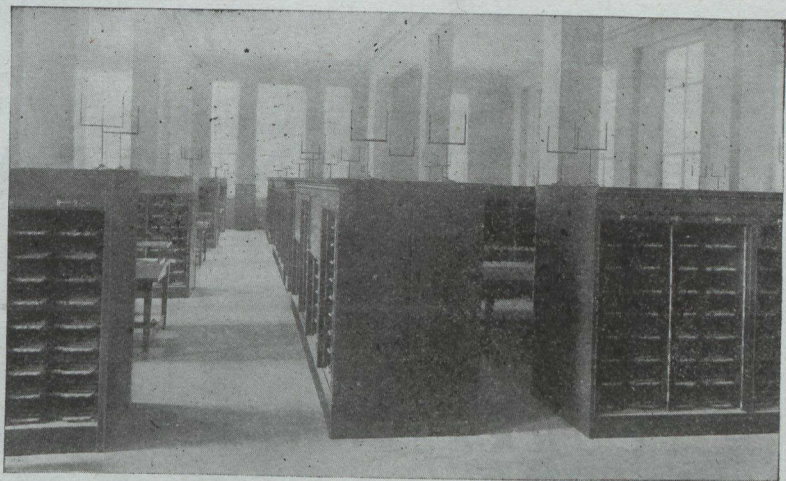
This interior view showing part of the "Office Specialty" Steel installation in Toronto Registry Office, shows a wide variety of equipment in use. Stacks with roller shelves for books (in front of which are Sliding Curtains); Reference Tables, Trucks, and Document Files.
