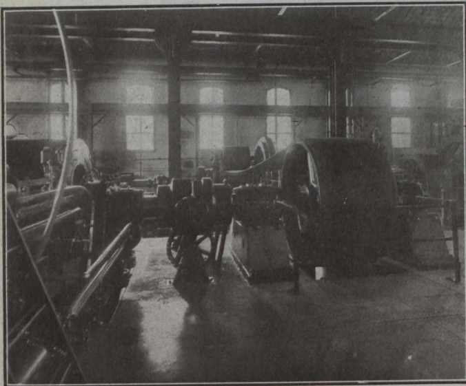
Shaft Extension to Gas Engine, For Driving Belted Unit. Photo, July 26th, 1917
