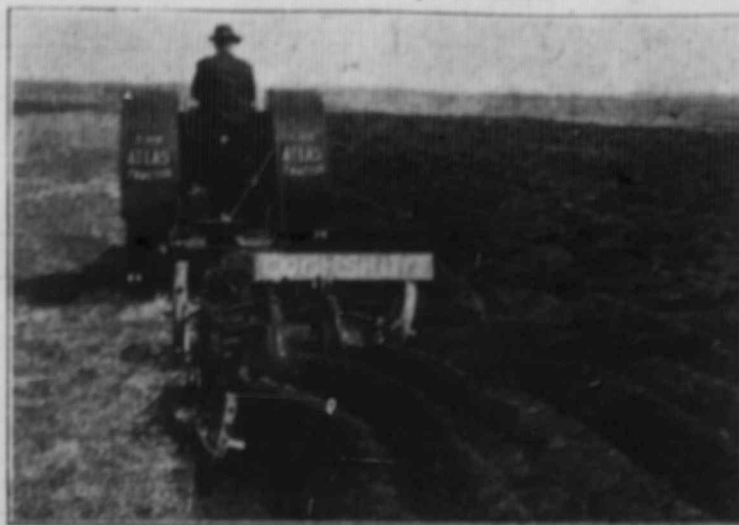
Taken from Actual photograph of the ATLAS TRACTOR pulling three 14-inch bottoms from six to eight inches deep through the toughest kind of virgin soil at the demonstration on Crescent Heights, Calgary, May 20th, 1918.
