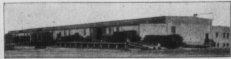
Distributing Warehouse, Elmwood, Winnipeg, of the United Grain Growers Limited. Size, 100 feet by 400 feet.
