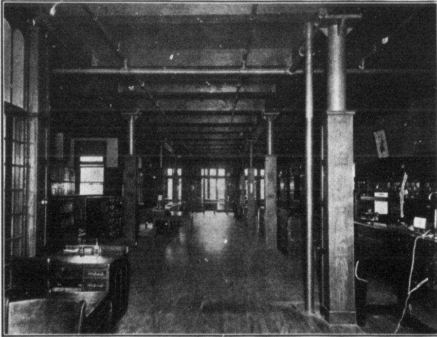
Fig. 1—Interior of office of Williams & Wilson, Montreal, Showing Catalogue Filing Cabinets to the left and Cupboards for Reserve Catalogues Built to the Wall
