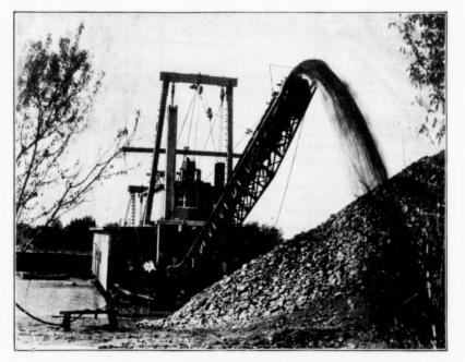
A BELT CONVEYOR ON DREDGE IN OPERATION,
