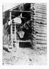
UPPER LOADING STATION - SHOWING TRIGGER AND GENERAL CONSTRUCTION OF BUCKET.
