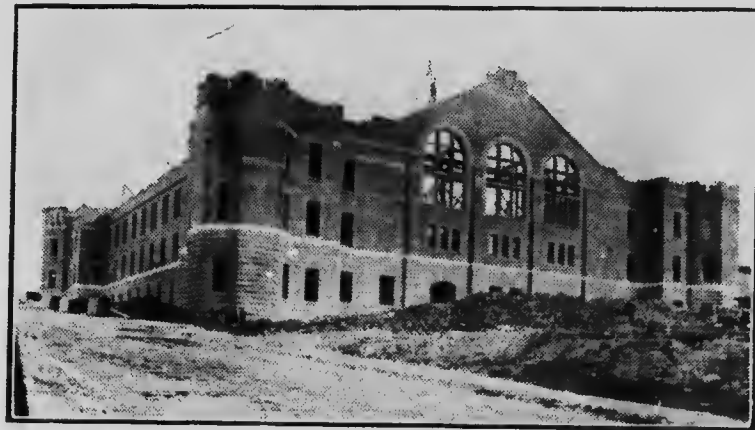
Most Modern Armory and Drill Hall in Lower Canada nearing completion. Estimated cost, $250,000.
