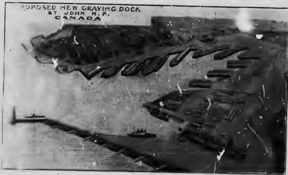
Harbor Works and Dry Dock under course of construction in Courtenay Bay by Norton-Griffiths & Co. Present Contract, $11,000,000. Estimated cost of completed work, $30,000,000.
