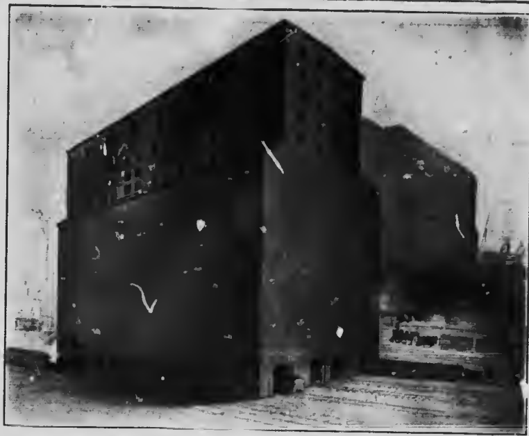
Concrete Elevator of a million bushels capacity under construction for the C. P. R. Estimated cost, $500,000.
