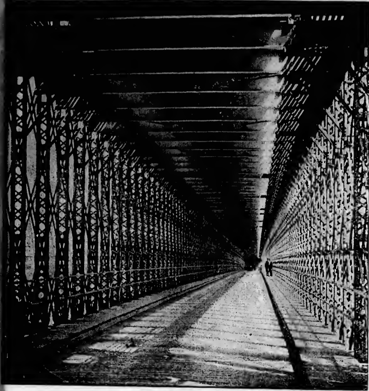
SUSPENSION BRIDGE ROADWAY.
