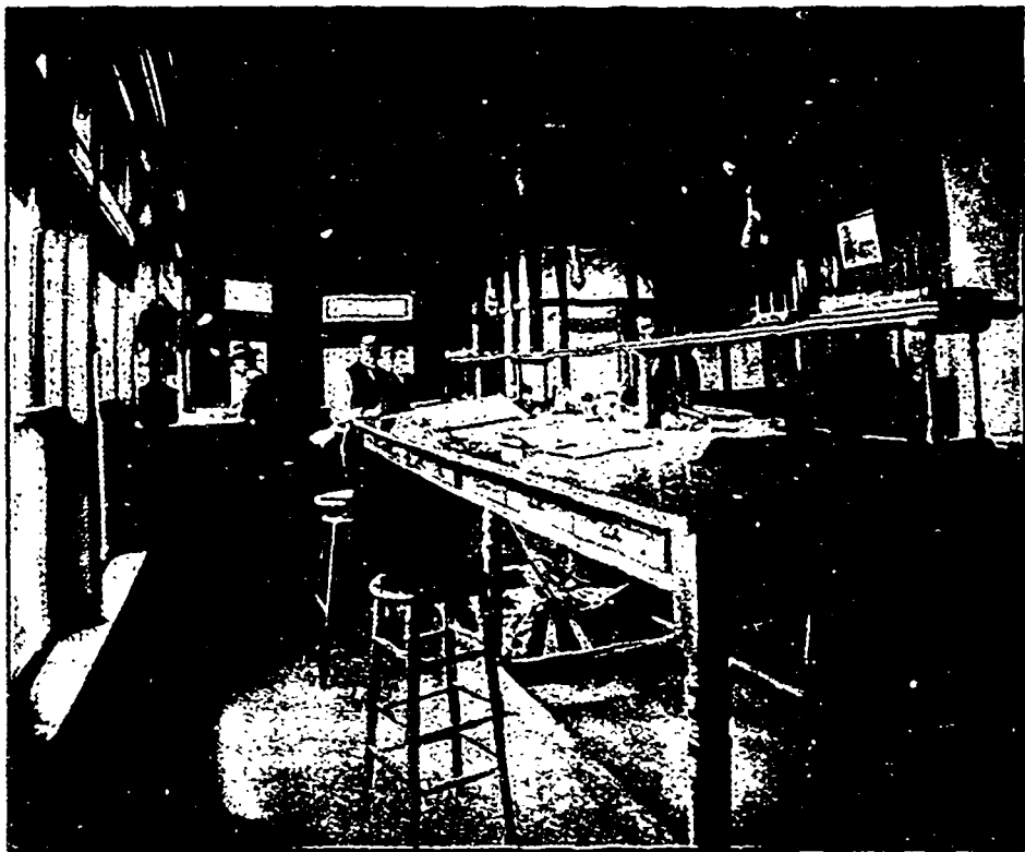
D. E. SPRAGUE—INTERIOR VIEW OF OFFICE.
