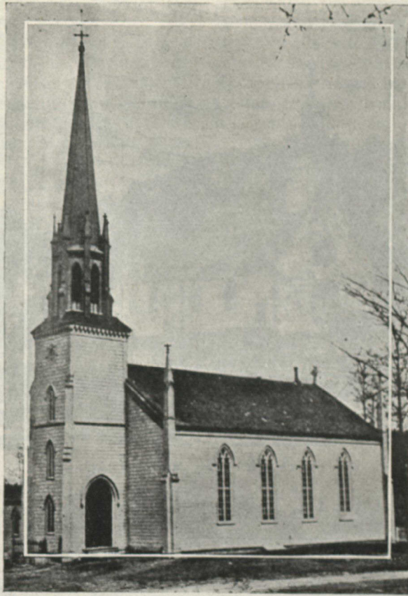
Old Trinity Church, Kingston, New Brunswick. It was built by United Empire Loyalists
