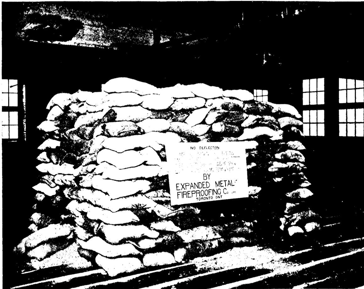
Floor Test. Mail Job Printing Co.'s Building, Toronto. Messrs. Sproatt & Rolph, Architects. Area loaded, 9 ft. by 11 ft. Weight of load, 32 tons, with NO DEFLECTION. The EXPANDED METAL SYSTEM of Concrete Reinforcement was used throughout in this Building.
