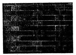
Fig. 7.—Another example of the double stretcher Flemish bond, only here the mortar joints are much thinner, being but oneeighth of an inch in thickness and slightly raked-out. The bricks used are  $8 \times 2!_2 \times 3\%$  inches in size, and of a rough texture; the stretchers being of dark clear red, and the headers of a brown blue color.
