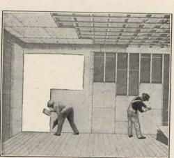
Method of applying Sackett Boards to Walls and Ceilings.
