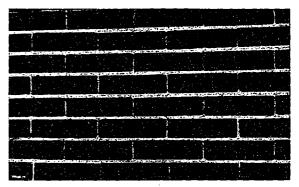
Fig. 9.—A wall of brick of ordinary s.ze, laid up in a running bond with the conventional 36 inch, raked, white joints. The color scheme, however, is noteworthy, the effect being produced with bricks of clear red, and reds with finished edges.
