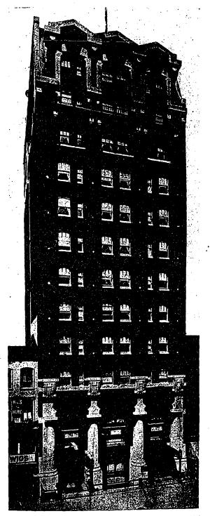
Fig. 4.—Hotel building of attractive design, the facade of which is built of red pressed brick with blue toned bricks for trimmings. These are laid up in the ordinary Flemish bond with white raked-out mortar joints of an appropriate thickness.
