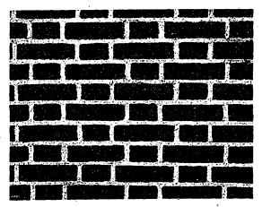
Fig. 6.—A wall of "tapestry" brick,  $8 \times 2^{1/2} \times 3^{3/4}$  inches in size, in Flemish bond and five-eighths of an inch struck mortar joints of white. All stretchers are of dark blue, while the headers are of medium red, to overcome the non-actinic properties of red and blue. This effect is a reversal of what is apparently the darker brick into the lighter, and vice versa.
