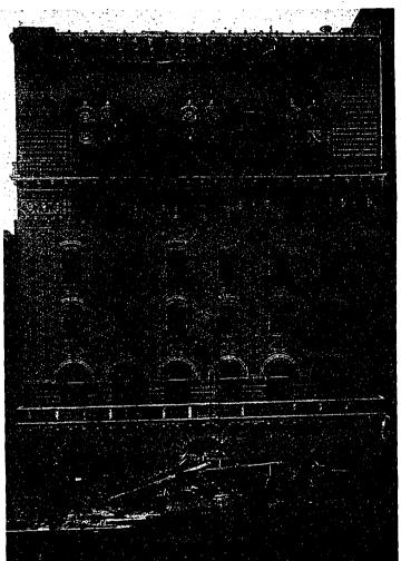
Fig. 1.—Facade of Club Building, showing an interesting treatment in diaper work. The bricks,  $12 \times 2^{1/2} \times 4$  inches in size, and of a rough texture, are laid up with a gray raked mortar joint, three-quarters of an inch in thickness, the bond being of a special character. The color tones are a soft warm gray tinged with brown, and white headers and special moulded bricks, on a smooth brown ground.
