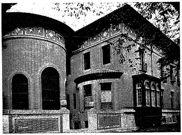
Fig. 2.—Brick residence in which the effect of the double stretcher Flemish bond and large horizontal mortar joints can be seen. The size of the bricks, which are of medium and dark shades, are  $8\% \times 17\% \times 31\%$  inches, and the vertical joints are narrower than those which run horizontally, the latter being 11/3 inch in thickness. The pattern of belt course beneath the eaves is particularly note-worthy.
