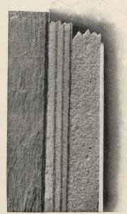
Sectional View (full size) of Sackett Plaster Board, applied to Wooden Stud, with ¾-inch grounds.
