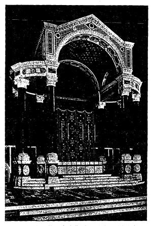
The Baldachino, New Catholic Cathedral at Westminster, London. An exquisite canopy of white marble, carved, panelied and inlaid with lapis-lazuli, and supported by eight monolith marble columns. The Altar beneath is a solid block of granite weighing fourteen tons. Every marble column in the building is a monolith. Mr. John Francis Bentley, Architect.
