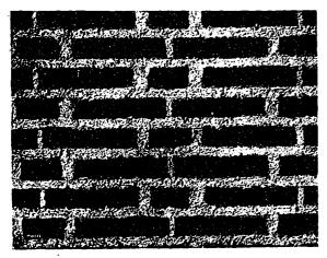
Fig. 8.—Although the bond is identical with that shown in the preceding illustration, in this case the joints, which are white and cut rough and flush, are 1/4 inches in thickness; while the brick itself is  $9 \times 2 \times 334$  inches in dimensions. Here the stretchers are gray and light brown, while the headers vary from gray and light to dark brown.
