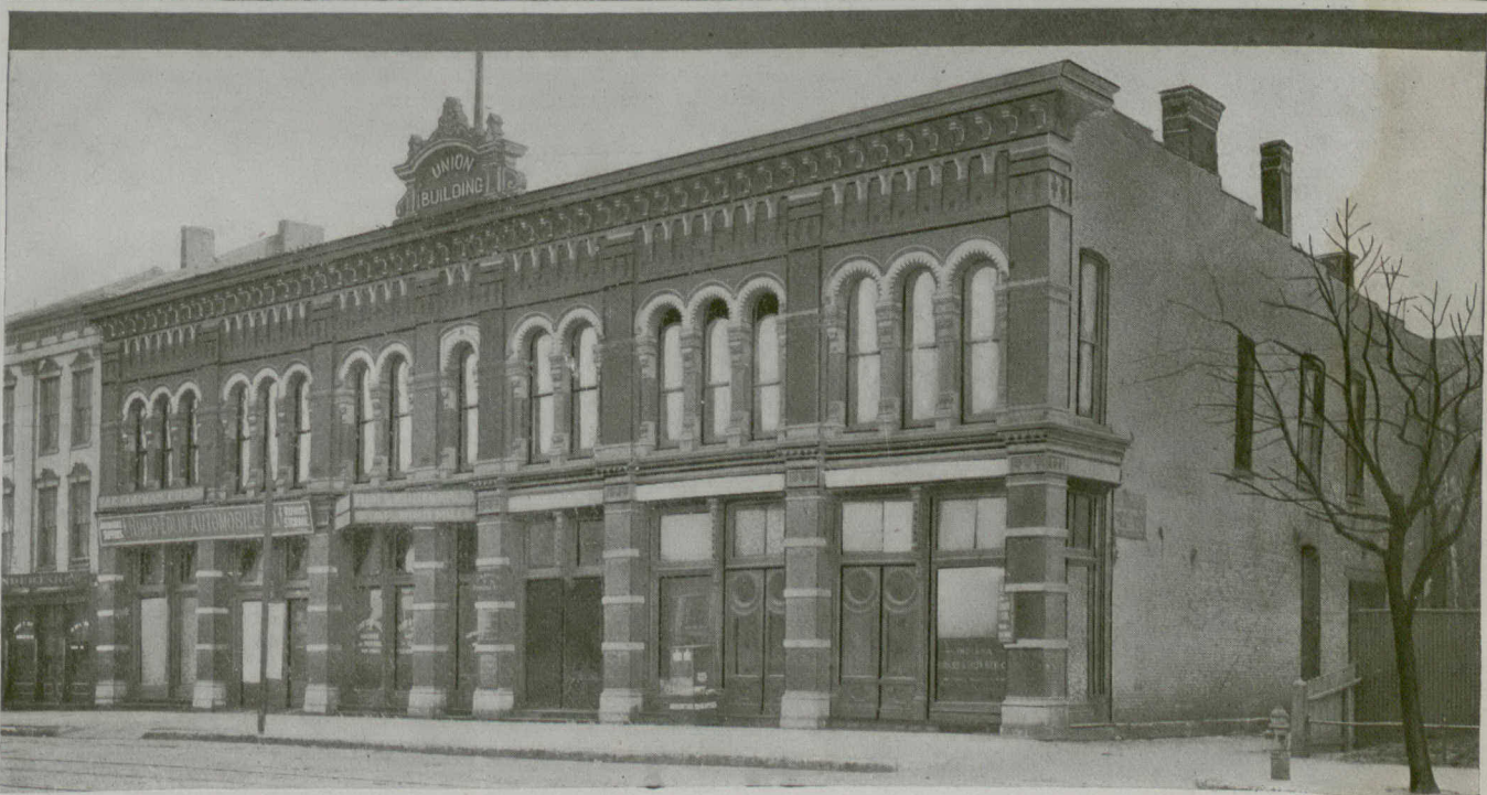
UNION BUILDING, INDIANAPOLIS, IND., ROOFED ALONG THE LINES OF THE BARRETT SPECIFICATION OVER 20 YEARS AGO.
