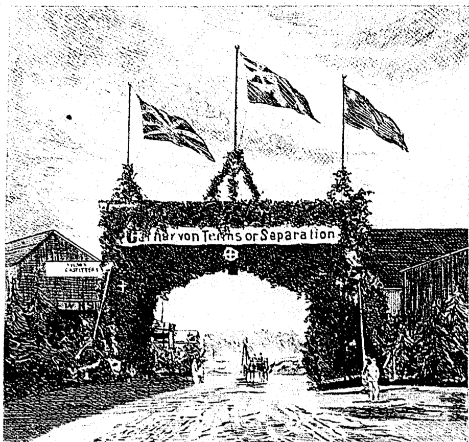
THE FORT STREET ARCH, LOOKING EAST.
