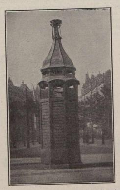
Fig. 7.—Superstructure for Ventilating a Trunk Sewer in Dresden. (The dome is equipped with selfrecording rain gauges.)
