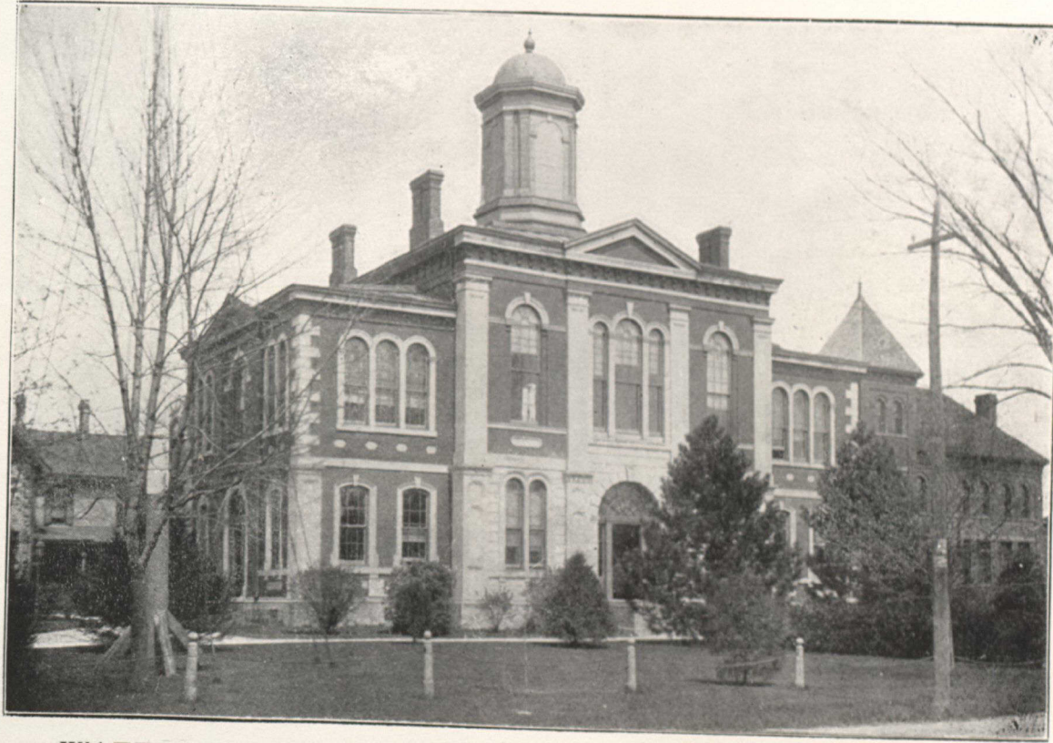
WATERLOO COUNTY PUBLIC BUILDINGS, BERLIN.
