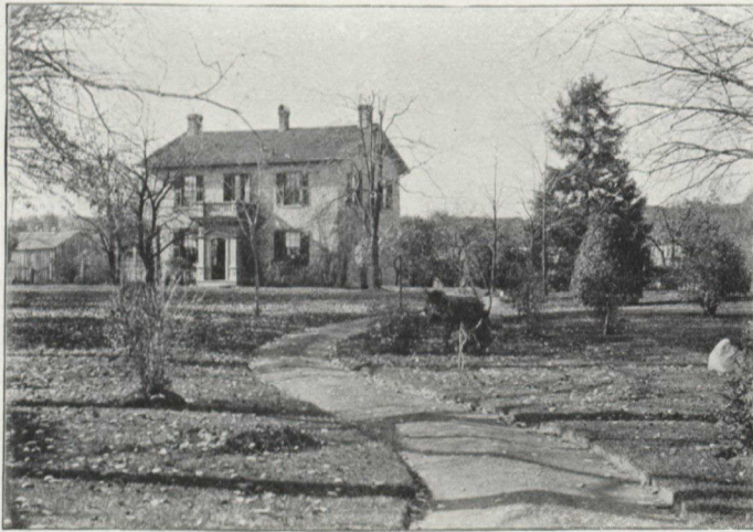
RESIDENCE OF ADAM WARNOCK, ST. ANDREW'S ST.
