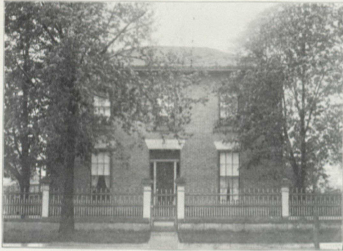
RESIDENCE OF MRS. ALLEN, MARKET ST.
