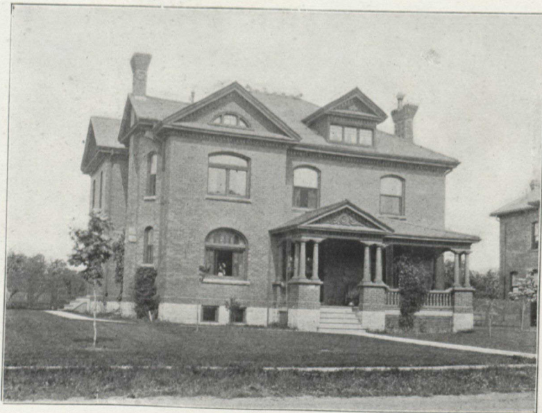
RESIDENCE OF R. STRUTHERS, LANSDOWNE AVE.
