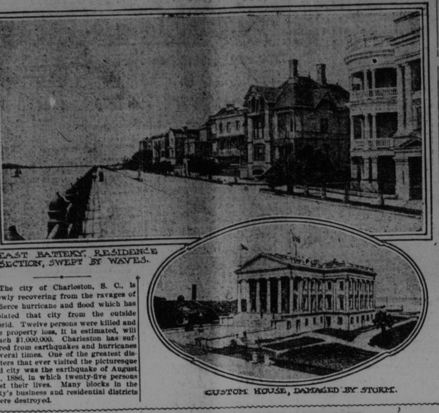
CUSTOM HOUSE, DAMAGED BY STORM.
