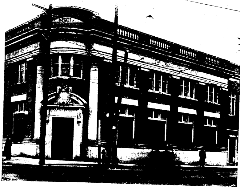
BANK OF OTTAWA, BROADVIEW AND GERRARD, TORONTO. John M. Lyle, Architect. C. A. Scott, Mason Contractor.
