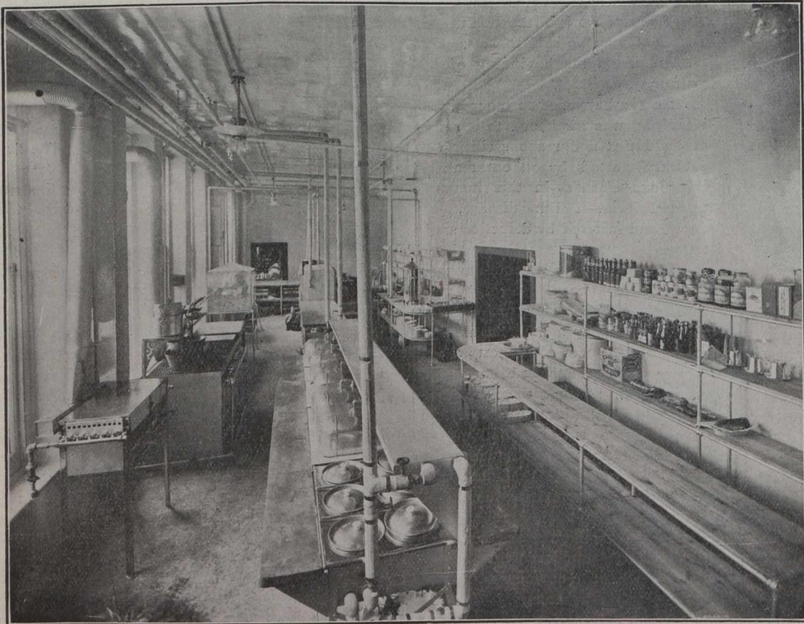
**Sanitary Kitchen of Grill Room, T. Eaton Company, Smooth Walls and Floors. Note Gas Pipe Fittings and Simple Tops For Same, Easily Removed for Cleaning, all Designed by the Food Inspectors.**
