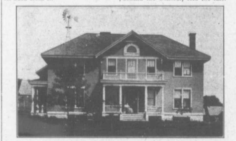
The commodious and comfortable farm home of Mr. J. W. Suddard, Frontenac County, Ont. Note the interior plans published on the following pages.
