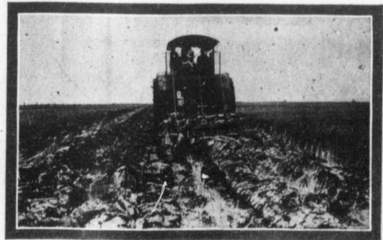
The Hart-Parr 15-30 Kerosene Tractor pulling a Six Bottom J.I. Case Engine Gang in the Plow Test.
