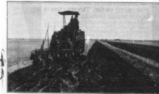
The Rumely 6 bottom engine gang in the Winnipeg Plow Competition. Note the evenness of the back furrow ridge.
