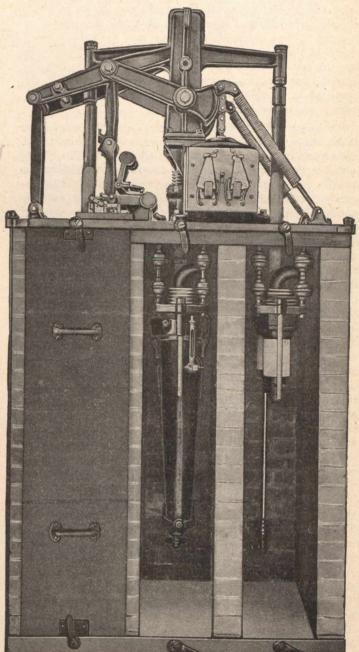
View of a Westinghouse, electrically operated, automatic, oil-break circuit<sup>+</sup> breaker, showing the left-hand compartment closed by an iron door, the oil tank sus<sup>-</sup> pended in the middle compartment, and the right-hand compartment without the oil<sup>-</sup> tank. The over-load relay is just above the second brick pier from the right, and the tripping device just above the third pier.
