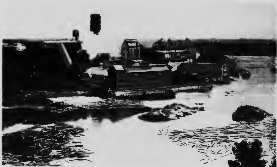
Laurentide Mills, Grand Mere. New Turbines 100 000 h.-p. single runner
