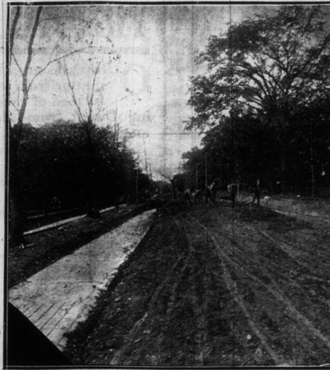
CIVIC IMPROVEMENTS AT GALLOW'S HILL. Workmen lowering the grade of road, after the laying of new concrete walk.
