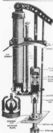
The sectional cut shows why The Spramotor Hand Sprayer is so effective, simple and durable. It will last as long as required for painting, white-washing, orchard, potato, and mustard spraying. There are more Spramotors in use in Canada than all others combined. It has agitator, which thoroughly mixes the paint or chemicals before they are applied, which acts independently of the motor. It has brass independent ball valves, which remain tight in use. The plunger has stood ten years' test.
