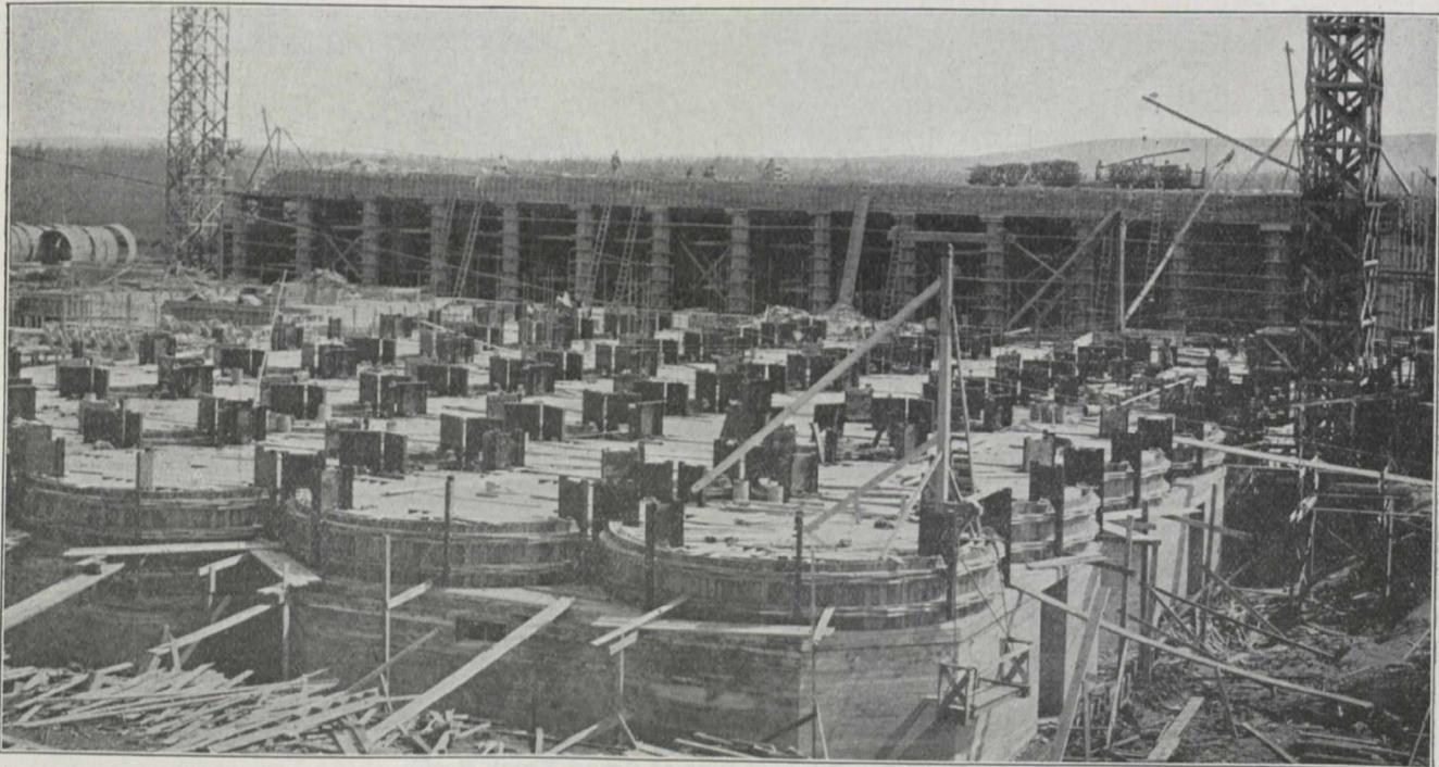
Fig. 2. Foundation and Substructure Grand Trunk Pacific Elevator, Fort William, Ont.
