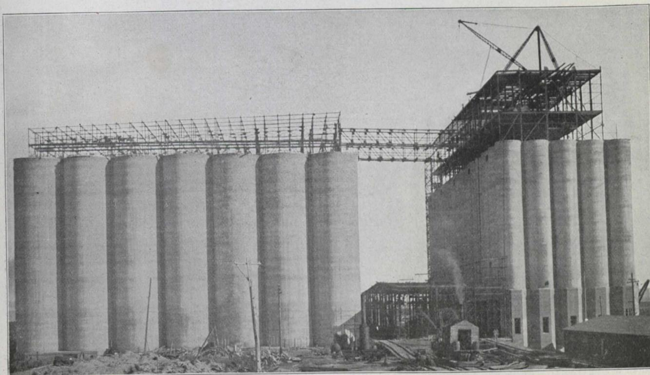
Fig. 3. Completed Bins and Steel Frames of Track Shed and Cupolas, Grand Trunk Pacific Elevators, Fort William, Ont.
