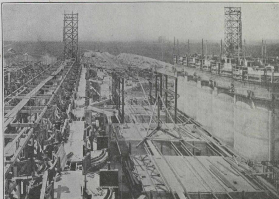
Fig. 1. Receiving Pits and Bins of Grand Trunk Pacific Elevator in Course of Construction.
