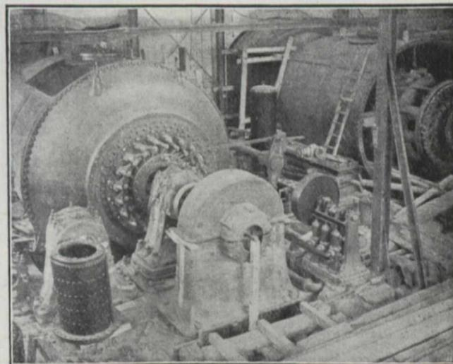
Fig. 4.—View of Turbine During Erection.
