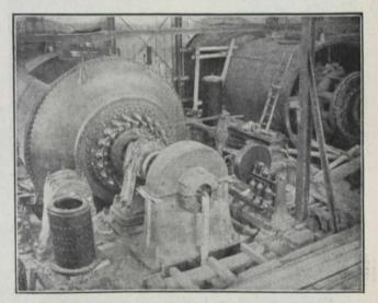
Fig. 4.-View of Turbine During Erection,
