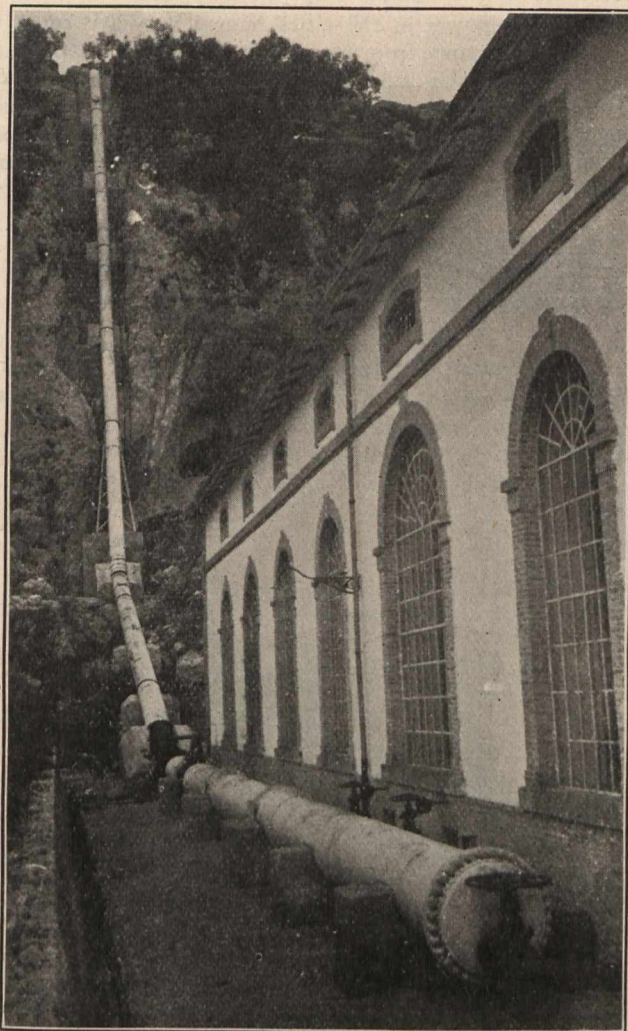
Fig. 6.—Olevano Station: Penstock 40-inch Diameter.
