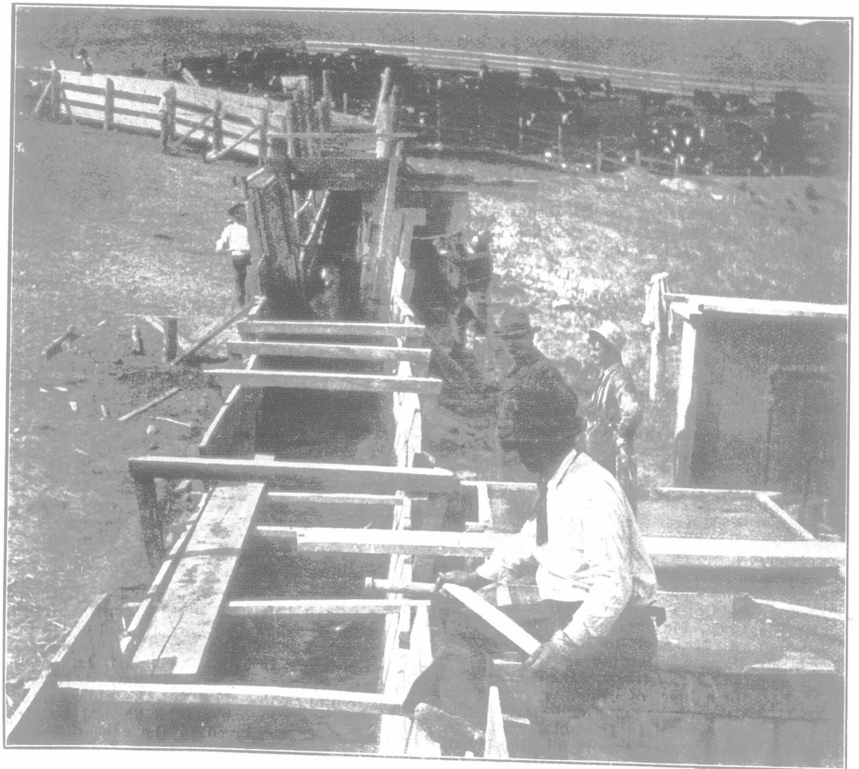
Through the Dip at Gleichen, Alta.
