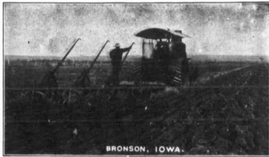
A Hart-Parr Gas Tractor Pulling an 8 Bottom John Deere Engine Gang
