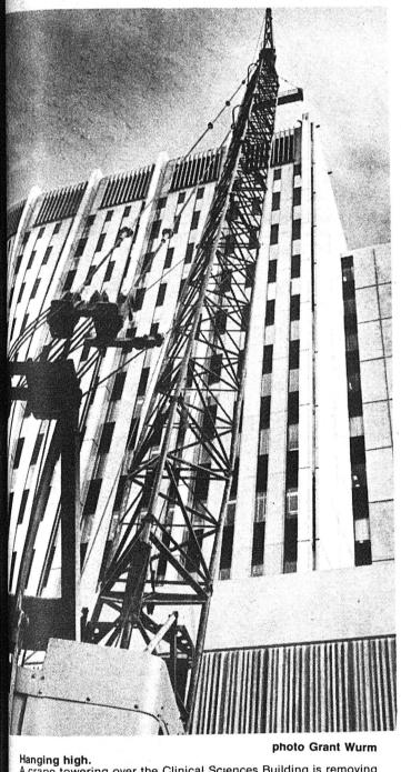
A crane towering over the Clinical Sciences Building is removing Merior bidg. facing which was loosened last fall in high winds. Meliminary examination, involving removal of 12 to 15 slabs, will cost \$0,000 — if the whole wall must be replaced, \$1.5 million.
