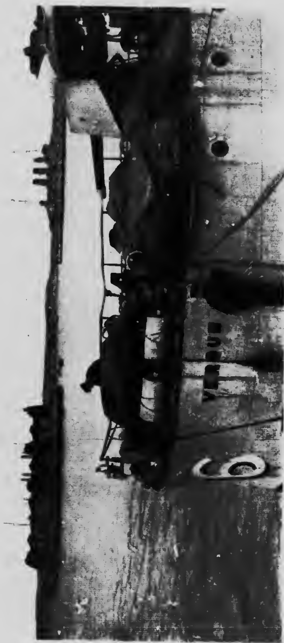
FLOATING DOCK FOR LIFTING SUBMARINES IN KIEL HARBOR
