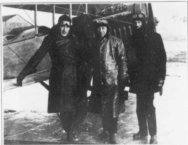
TEST OF FIRST C.A.L. MACHINE.
