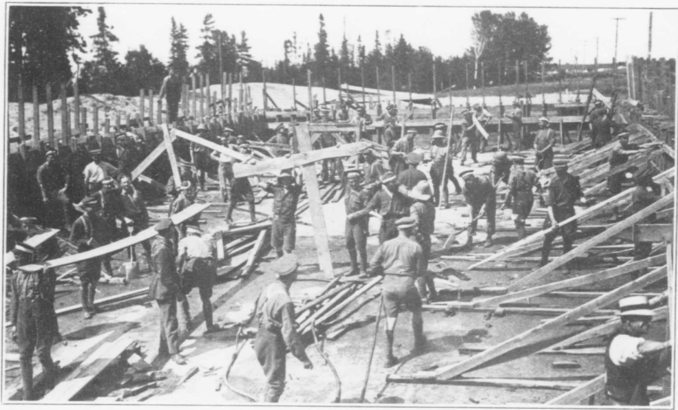
CONSTRUCTION OF SWIMMING POOL, CAMP BORDEN. (Under Direction of Aviation Department.)
