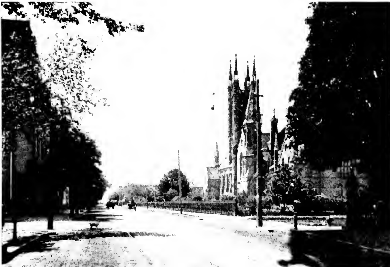
CORNER OF SHUTER AND CHURCH STREETS, TORONTO.
