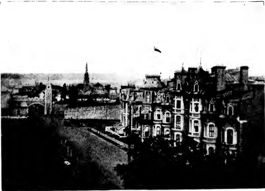
GRANDE ALLÉE AND ST. LOUIS GATE, QUEBEC.
