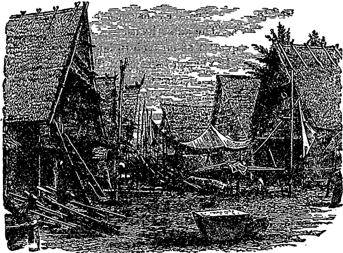
STREET ARCHITECTURE, DOBBO, ARRU ISLANDS.
