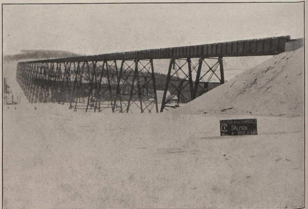
Little Salmon River Viaduct, New Brunswick. Mile 184 from Moncton. Length, 3,918 ft. Height, 200 ft. Tons Steel, 6,995.
