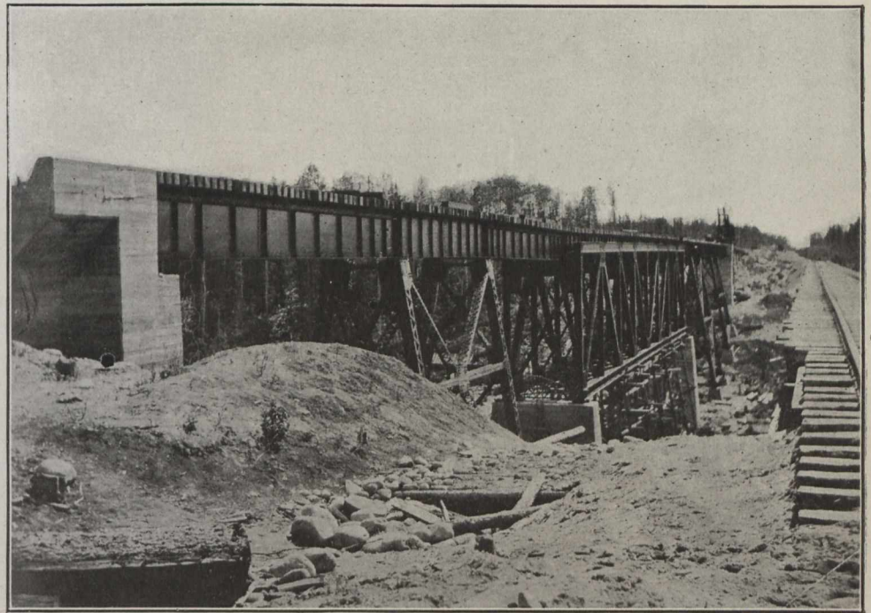
Frederickhouse River Bridge, Ontario. Mile 1034 from Moncton. Length, 622 ft. Height, 78 ft. Tons Steel, 670.
