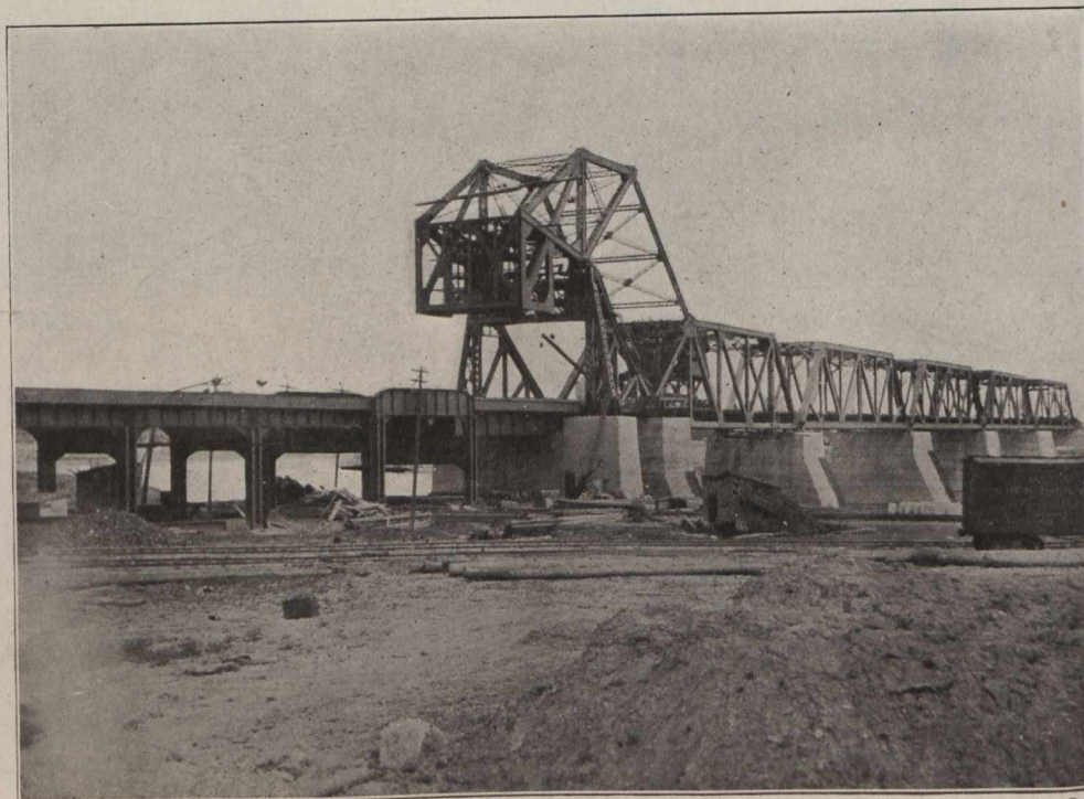
Red River Bridge, Winnipeg. Mile 1,804 from Moncton. (Strauss Bascule Lift Span of 129 ft. 6 in.)
