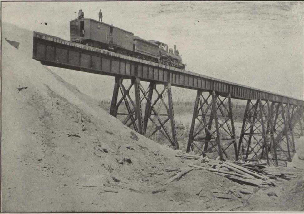
Canaan River Bridge, New Brunswick. Mile 21.6 from Moncton. Length, 532 ft. Height, 84 ft. Tons Steel, 424.
