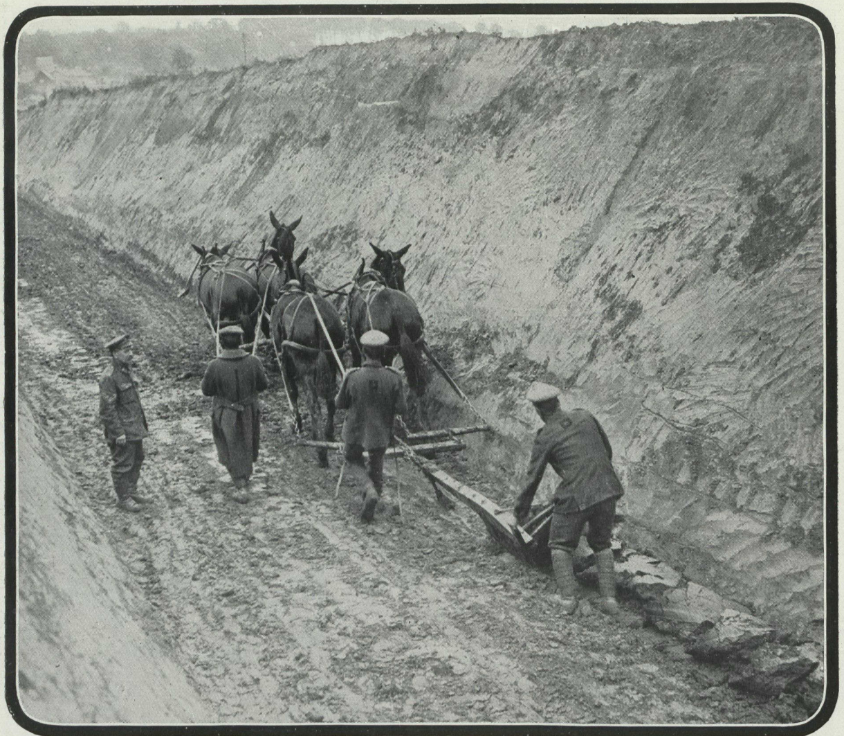
Light Railway construction troops ploughing up the earth which the drag "scrapers," drawn by mules, carry away for "dumping"
