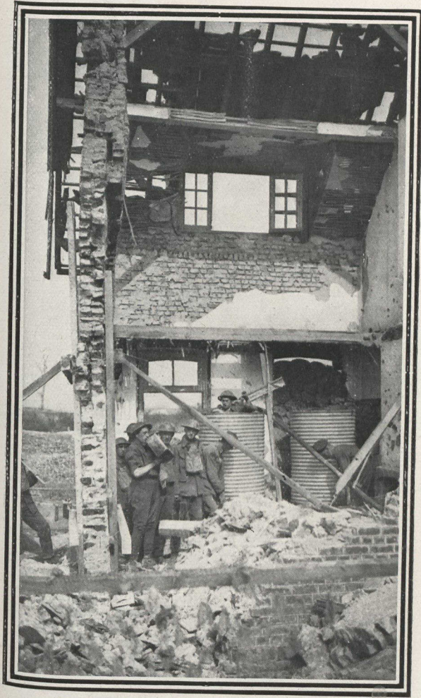
Battered shelter for water tanks
