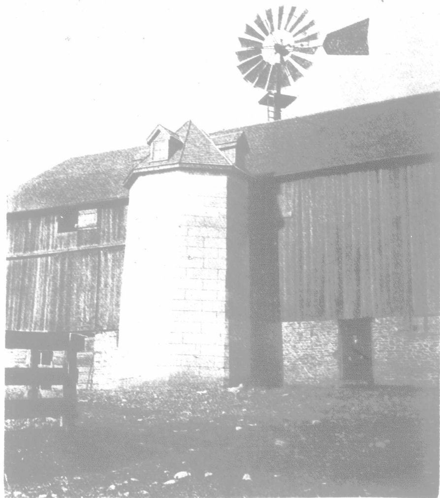
Farm of A. C. Pettit. Silo built with Battle's Thorold Cement. Dimensions 30 feet high and 12 feet in diameter. Driving-house floor 26 x 36 feet.
