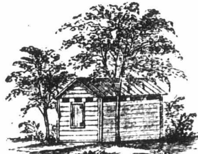
Fig. 1—Rough or Shanty Ice House, left open under the Eaves for Ventilation.
