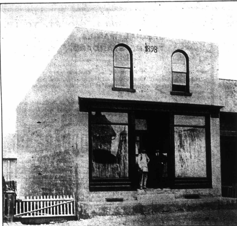
CONCRETE STORE OF W. F. FORREST, ATWOOD, ONT. Dimensions: 22 x 60 x 29 feet high. Built with Thorold Cement.
