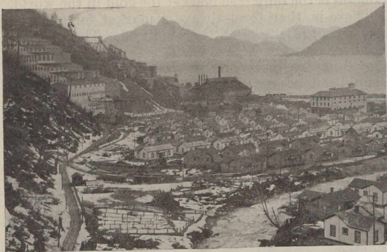
Mill, Bunkers, Store and Beach Town-sites, Britannia M. & S. Co., Britannia Beach, B. C.—Mill Produces 2,000,000 lbs. Copper per month.
